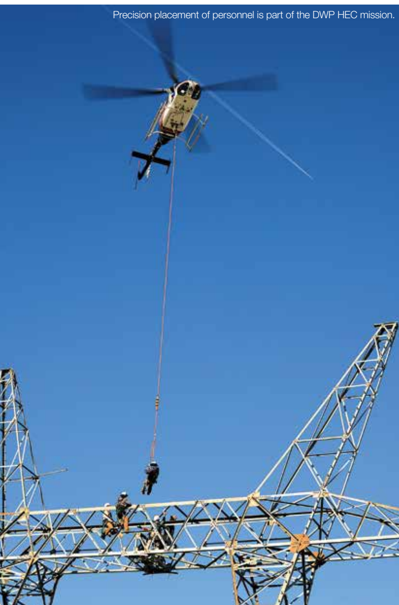
Dual hooks from Boost Systems are used for the human external cargo (HEC) operations.
