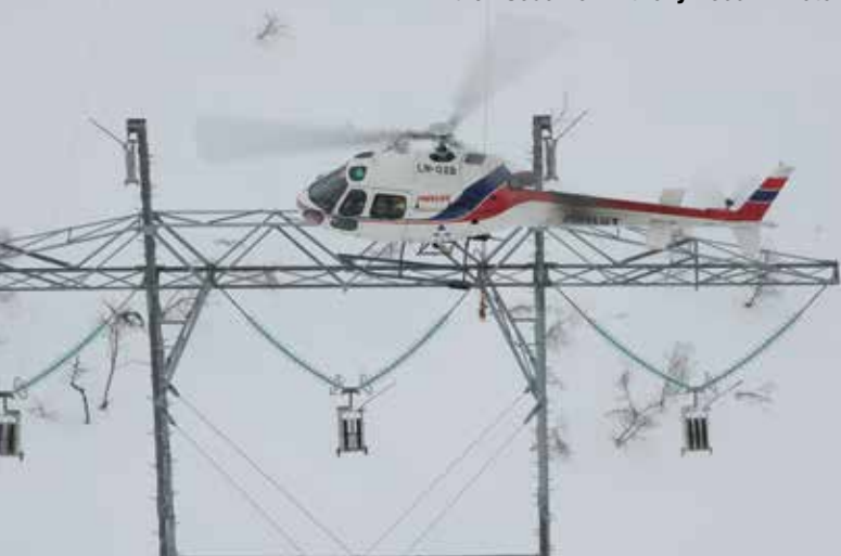
Airlift has become a specialist in constructing powerline towers, with the towers in Norway designed to meet the lifting and handling capabilities of the AS350 B3. Anthony Pecchi Photo
